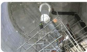
Wet and dry film thicknesses were tested with various gages throughout the project. Also done throughout, the crew members were sure to wear harnesses and lanyards when working from heights.
