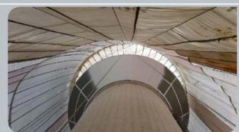
around the perimeter of the tank. On this project, there were a total of 54 outriggers installed. Then, to build the containment tree, the pulleys were welded around the center of the tank. The pulleys were used to run the cables to the top of the tank to allow the crew to winch the container to the top.
