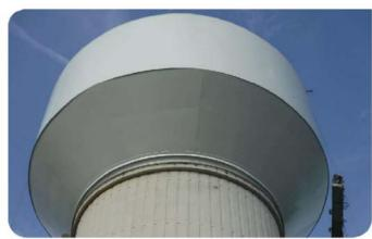
Despite delays with having welders add the exterior panels and stops throughout the job to avoid heat exhaustion, the Blastco crew got all prep work, coatings, and linings done. Maintenance achieved!
