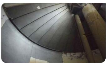
On the inside, surface prep included the use of AMASTEEL to achieve a NACE No. 2/Society for Protective Coatings (SSPC) Surface Preparation (SP) 10: Near-White Blast Cleaning, as well as dehumidifiers.
